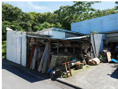
The entrance to Suga's studio, with its accumulation of overflowing outhouses constructed of scaffolding and corrugated plastic.
